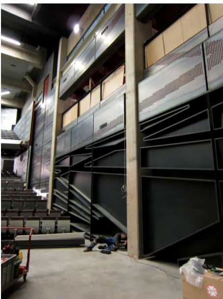
Figure 4. Sidewall diffuser structures
