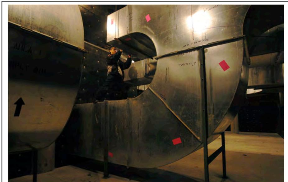
Figure 2. Kiyoshi Kuroiwa performing acoustic measurements in the plenum underneath Hammerson Hall at the Mississauga Living Arts Centre. Mr. Kuroiwa is holding a sound level meter but it is blocked from this view by the duct.
