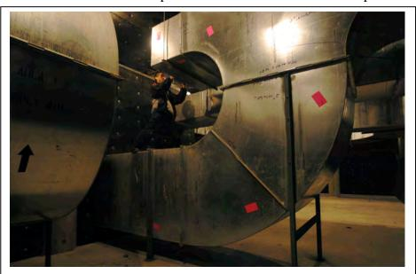
Figure 2. Kiyoshi Kuroiwa performing acoustic measurements in the plenum underneath Hammerson Hall at the Mississauga Living Arts Centre. Mr. Kuroiwa is holding a sound level meter but it is blocked from this view by the duct.
