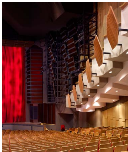
Figure 5. Zone 2 balcony fascia reflectors are seen in the foreground. Note how they progressively move toward the centre-line of the room. The Zone 1 proscenium reflectors are seen in the background.
